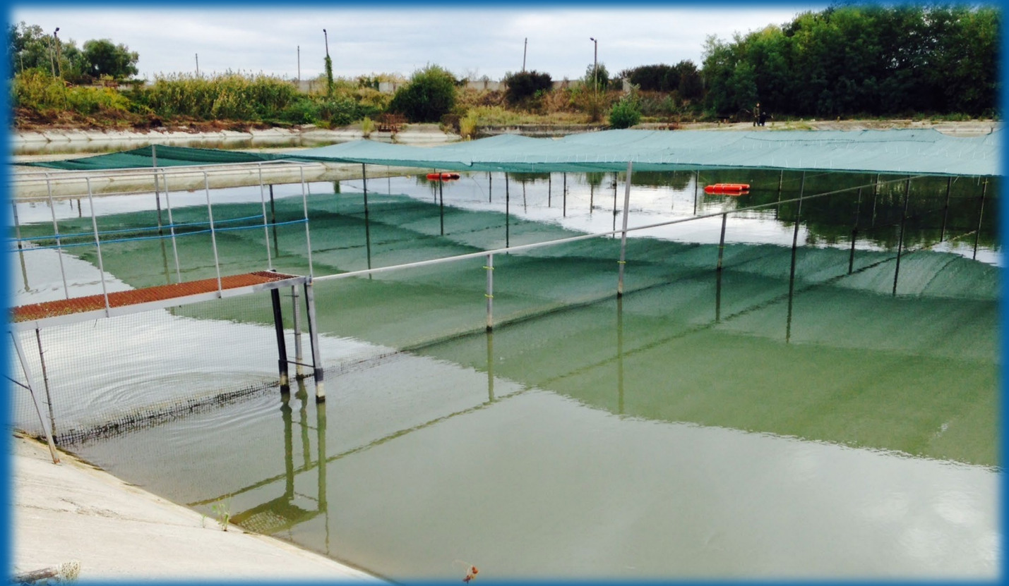
Open pond recirculation system
